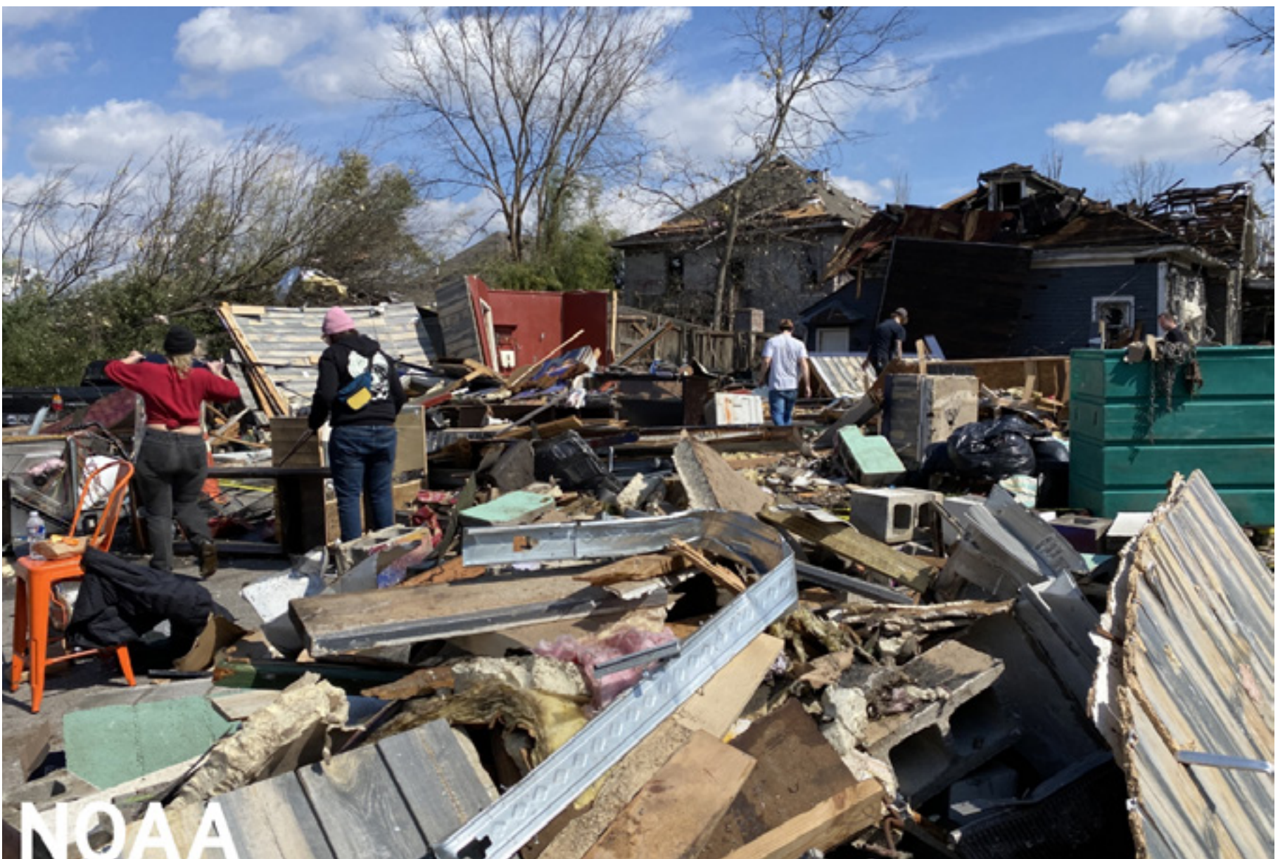
Heavy damage in East Nashville, Tennessee after tornadoes ripped through the region on March 3, 2020. Image credit: NOAA NWS.
